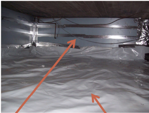
Repaired Wall Insulation
