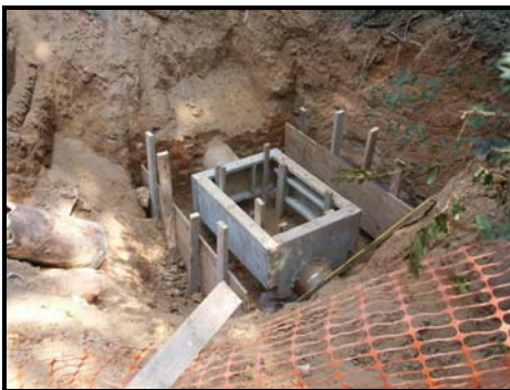
Figure 3a. Drain by-pass structure
