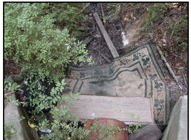
Figure 1b. Original Drain Outfall
