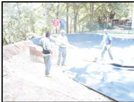
Figure 5a. Install fabric barrier
