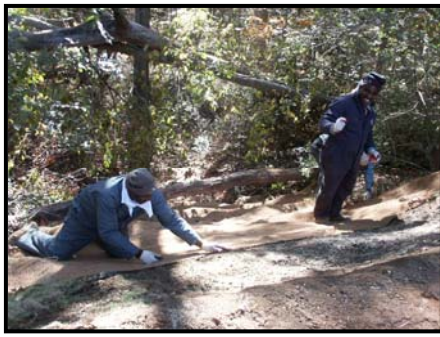
Figure 6b. Erosion fabric on berm
