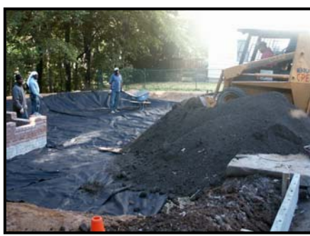
Figure 5b. Install soil mixture
