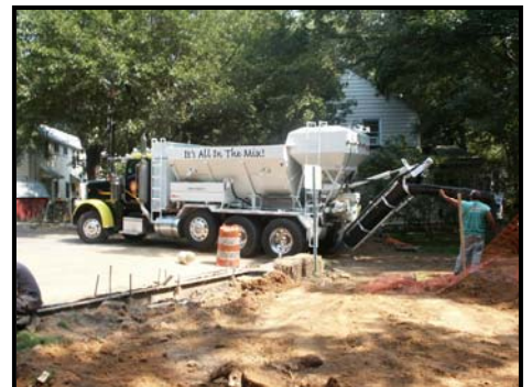
Figure 3c. Pouring parking curb
