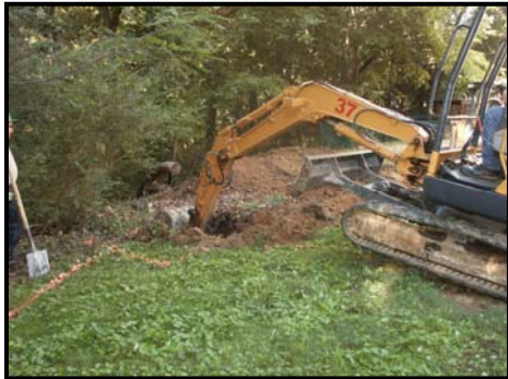
Figure 2a. Initial Excavation
