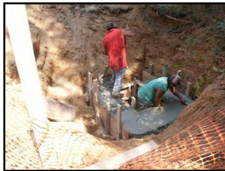
Figure 3b. Pouring by-pass
