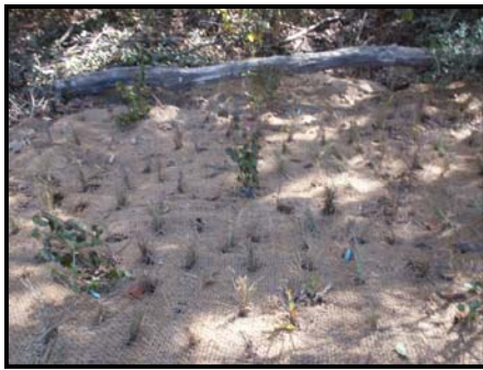
Figure 6c. Planted back slope
