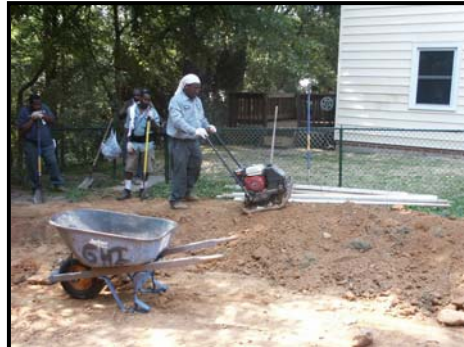
Figure 4b. Compacting berm
