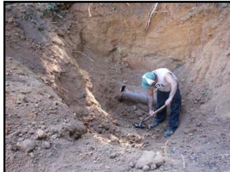
Figure 2b. Existing Drain Pipe
