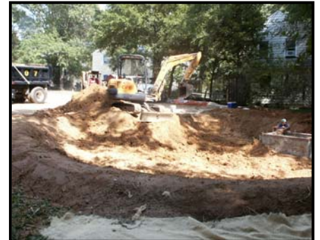
Figure 2c. Forming berm
